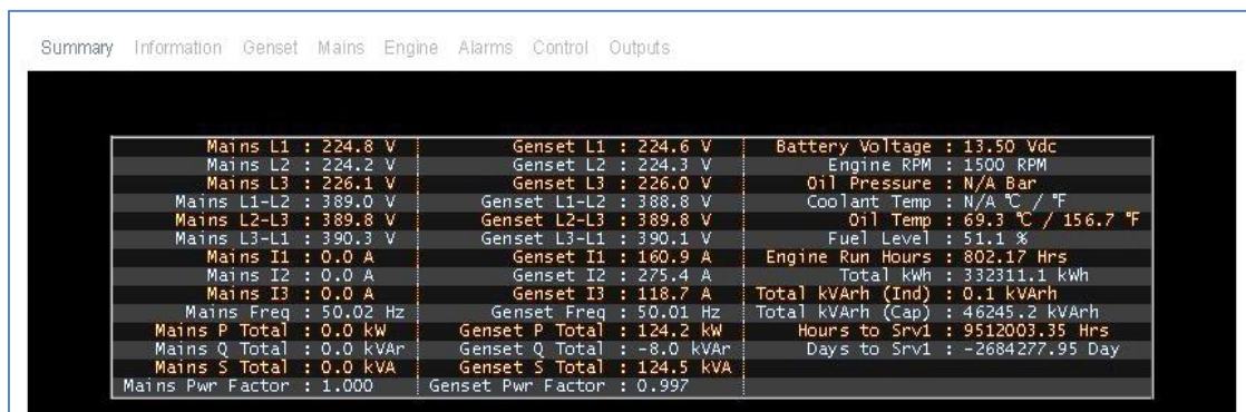
Real time monitoring
